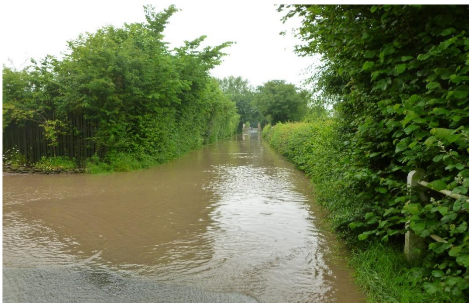
Fig.7: Kings Road, Orleton, October 2019 following 44.6mm of rain in 24hrs, taken from adjacent to Kings Road Severn Trent sewage pumping station looking towards B4362.
