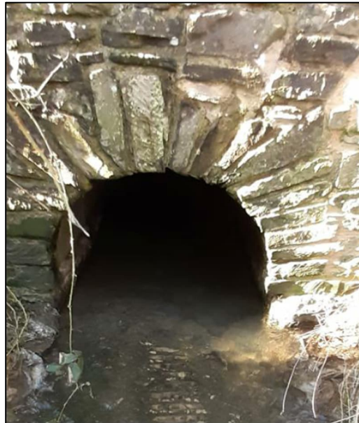
Figure -4: Downstream of B4361 Ashley Moore culvert, believed to be part of original field drainage
